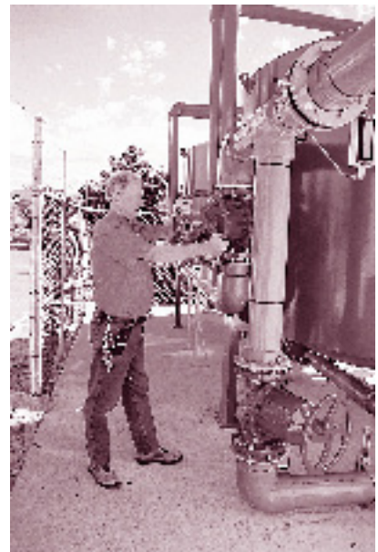
Figure 58 Working with new equipment
