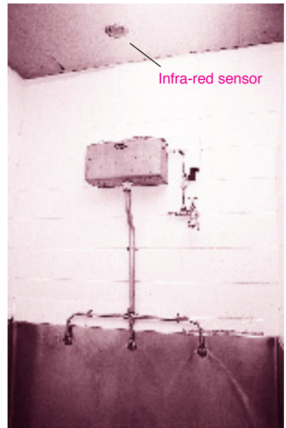
Figure 40 Installation of a Zip infra-red sensor urinal
