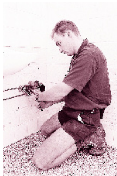
Figure 6 Stage 1 meter installation
