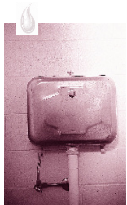
Figure 41 Stainless dual flush toilets were installed for students.
