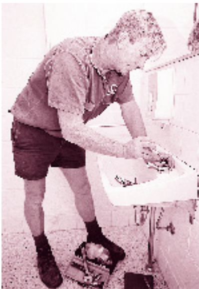
Figure 11 Fitting of water-saving equipment — Stage 2
